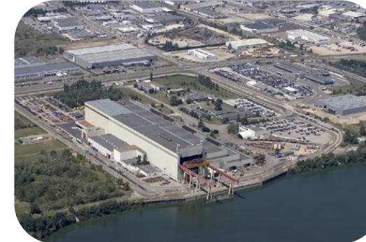
Chalon plant, upgraded and expanded
